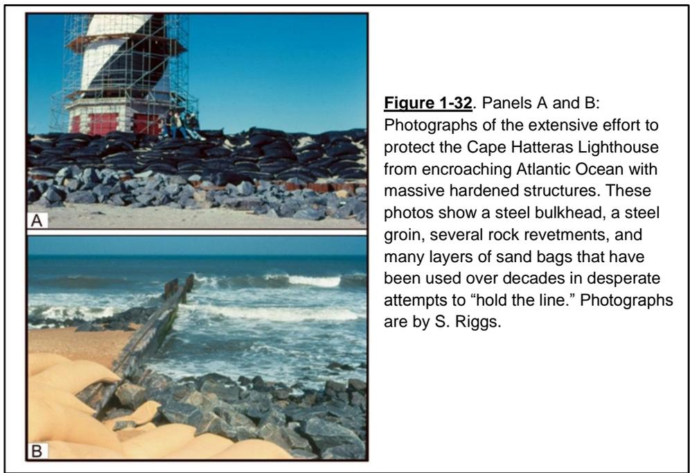
**Figure 1-32.** Panels A and B: Photographs of the extensive effort to protect the Cape Hatteras Lighthouse from encroaching Atlantic Ocean with massive hardened structures. These photos show a steel bulkhead, a steel groin, several rock revetments, and many layers of sand bags that have been used over decades in desperate attempts to “hold the line.” Photographs are by S. Riggs.
